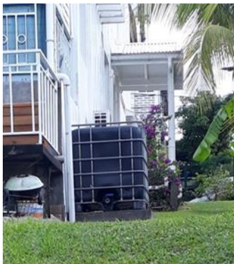
Figure 51 : cuve IBC opaque
