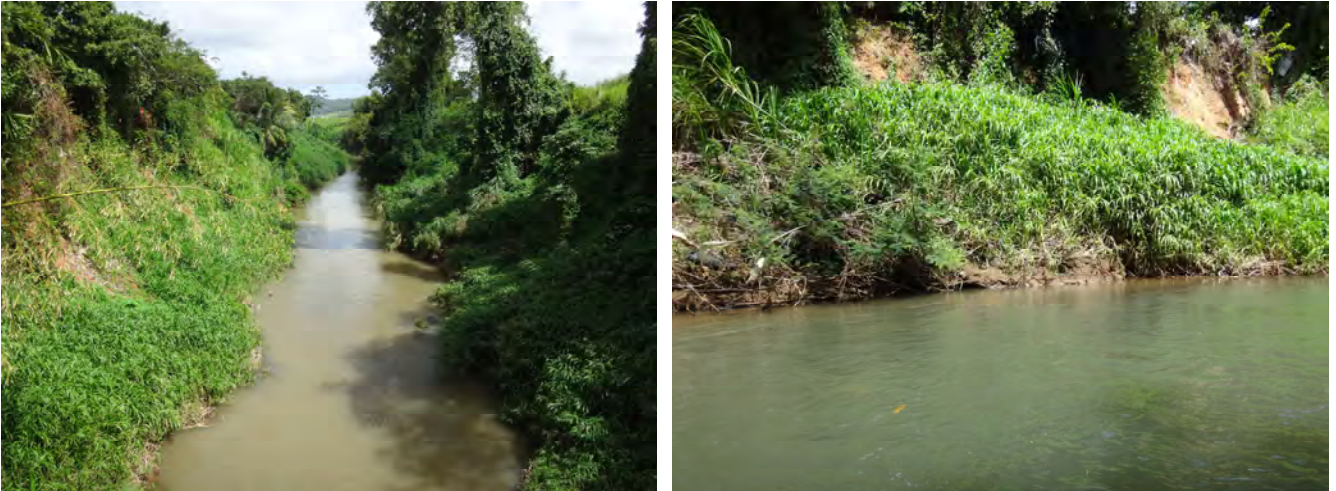
Figure 17 - Lézarde à Ressource - Station n°08541101 - 2018 - SCE
